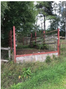
Cattle Loading Ramp
