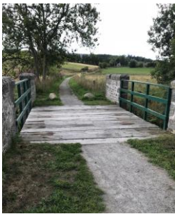
Learney Burn Bridge (good for pooh sticks)
